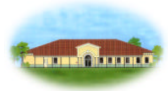
The Hope CommUnity Center 1016 North Park Avenue Apopka, Florida 32703
